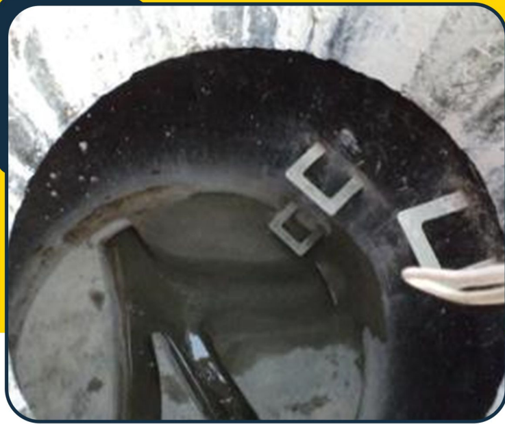
7 Complet Benching With Iron steps
