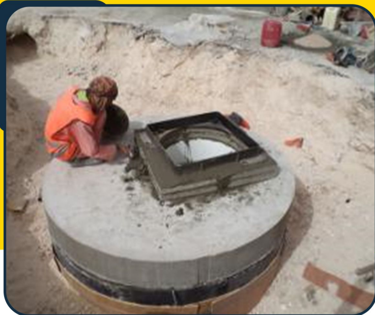
9 Installed Coverslab
