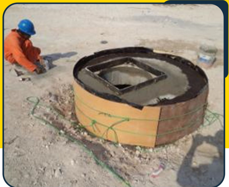
10 Installed Cover Frame with Concrete Haunch
