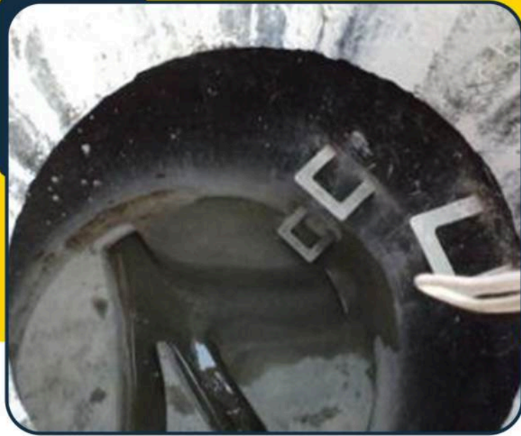
7 Complet Benching With Iron steps
