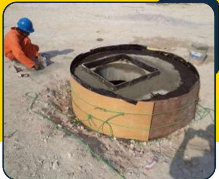
10 Installed Cover Frame with Concrete Haunch
